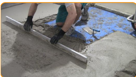
Build the screed
