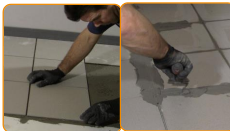
Install the floor finishing (ceramic or wood)
