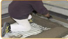
Install the reinforcement mesh (Ø 5 mm, net Apply the finishing on top of the screed and 200 mm) and build the screed (th. > 60 mm).
