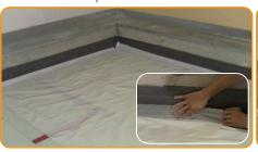
Apply a waterproof foil on the whole surface to protect the resilient layer.
