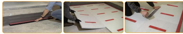
Install the adhesive strip Profyle Flat to the wall and the Side Highmat along the whole perimeter.
