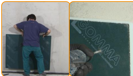
Place the panel on the right wall position and produce 5 holes per panel with the driller (one in the centre and one in the four corners)
