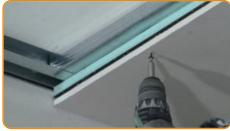
Fix the Rewall panel to the metal frame with Apply the plastic mesh tape in the gypsum 55 mm screws every 15 cm
