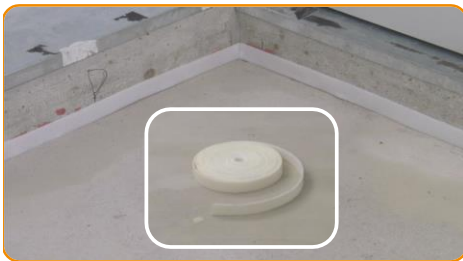
Fix the Profile Flat 5 around the bottom of the surrounding walls
