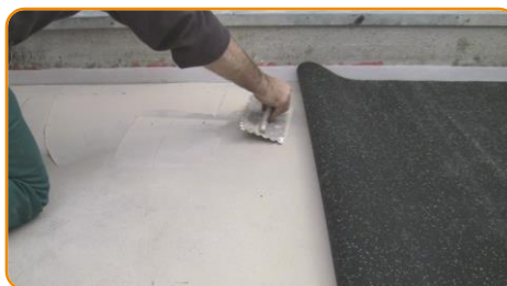
Spread a thin layer of adhesive onto the floor, then glue the Sylcer
