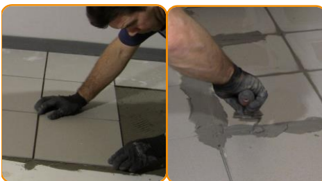
Install the floor finishing (ceramic or wood)
