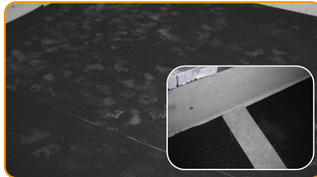
Install the acoustic mat with the textile facing up. Seal the joints with the Stik tape
