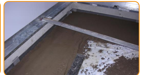
Build the screed
