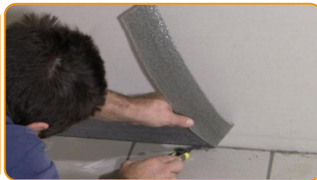
Cut the exceeding part of the edging strip
