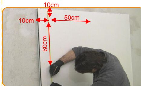
On each Rewall panel mark the holes points placed as per the drawing here shown
