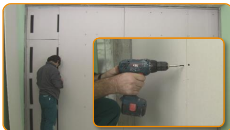
Fix the second gypsum board by gluing dots or screwing it on centre line and on the side borders with double thread screw. Offset
