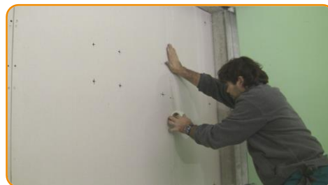
Apply the plastic mesh tape in the gypsum boards jointing lines
