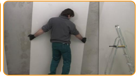
Apply the panel on the wall by forcing with homogeneous pressure.
