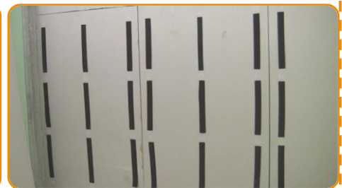
Apply the adhesive Syl strip between two nails
