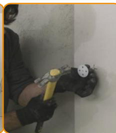
Proceed drilling the halls by a 10 mm driller and apply the nails
