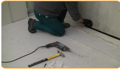
Lay the under wall strip
