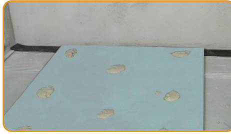
Apply the glue on the panel by spreading it on dots. (suggested glue Knauf Perfix)
