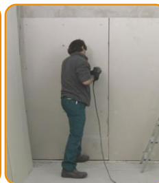
Proceed drilling the halls by a 10 mm driller and apply the nails
