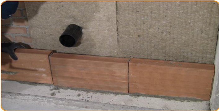
Start to built the wall
