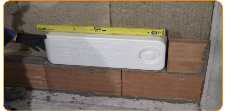
Lay on mortar the Sylencer
