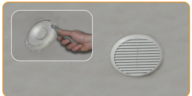
Cut or remove the cap and insert the grid in the hole of the Sylencer
