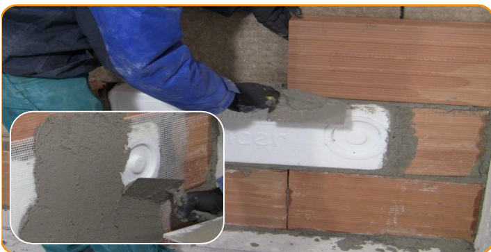
Build the wall around the Sylencer and plaster onto the product with a plastic mesh
