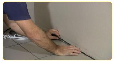
Remove the protective film and glue the strip along the perimeter Apply ceramic or wood baseboard to the wall above the Profyle Flat of the room 1
